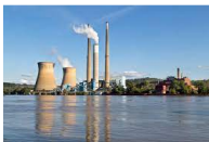
Power plant (kV's)
